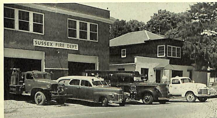
Fire Fighting Equipment
